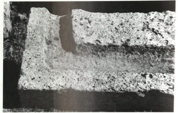
Fig. 8. End of the sponge gutter of the multi-seater of the North Service Building (26).
