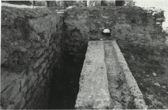
Fig. 7. Start of the sponge gutter in the multi-seater of the North Service Building (26) with hole for the supplying lead pipe.
