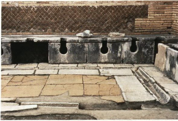
Fig. 2. Public toilet with marble seats, front plates and sponge gutter near the Forum Baths at Ostia.
