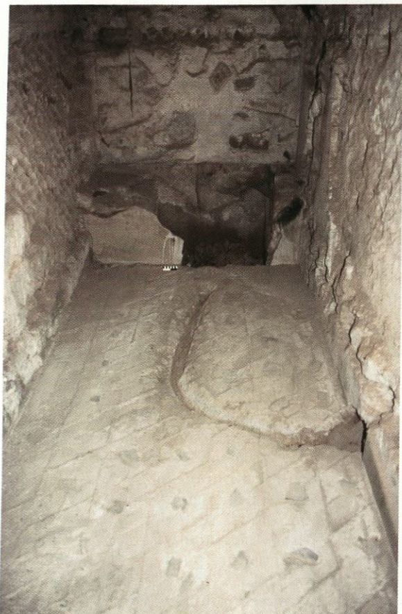
Fig. 11. Single-seater in the west wing of the Scenic Triclinium (40) with remains of marble seat and imprint of opus sectile floor. The groove indicates the position of the water pipe (photo R. Kragting).
